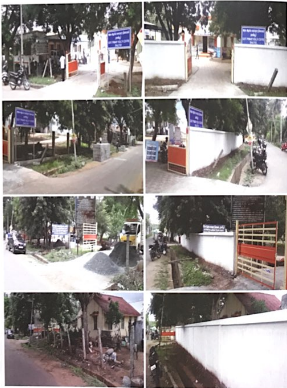
DHALIYUR Dhaliyur PHC Compound wall (Before & After)
