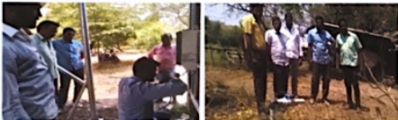
SOLAR FENCING ERECTION
