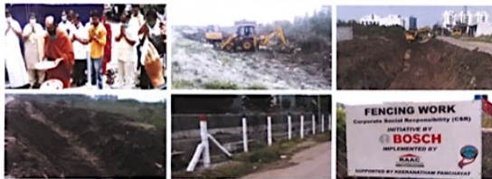
DESILTING OF THE WATER CHANNEL NEAR BOSCH NEIGHBOURHOOD
