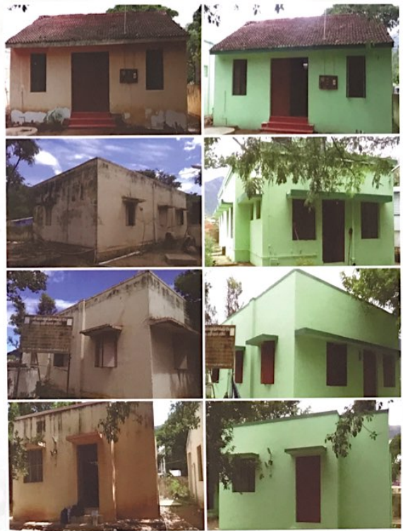
VEERAPANDI 24 Veerapandi PHC Painting Work & Electrical Work (Before & After)
